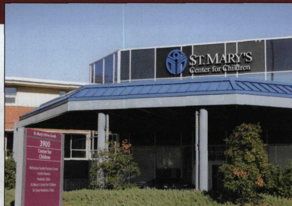
The exterior of St. Mary's Center for Children in Evansville, Ind.
