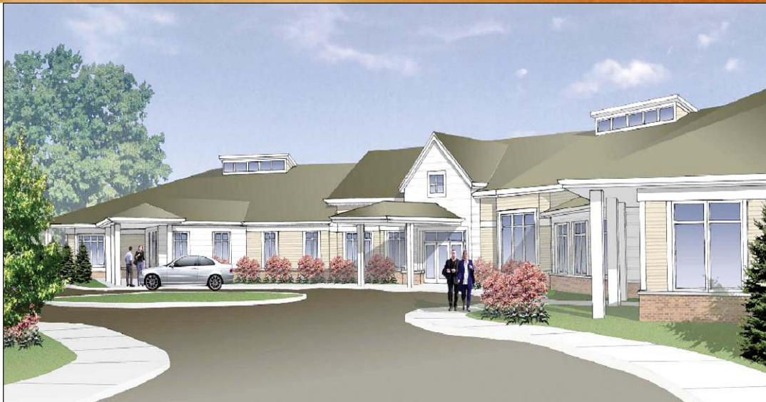
Exterior rendering of Evangelical Homes of Michigan's $12 million Memory Support Center, which includes "smart" residential units.
