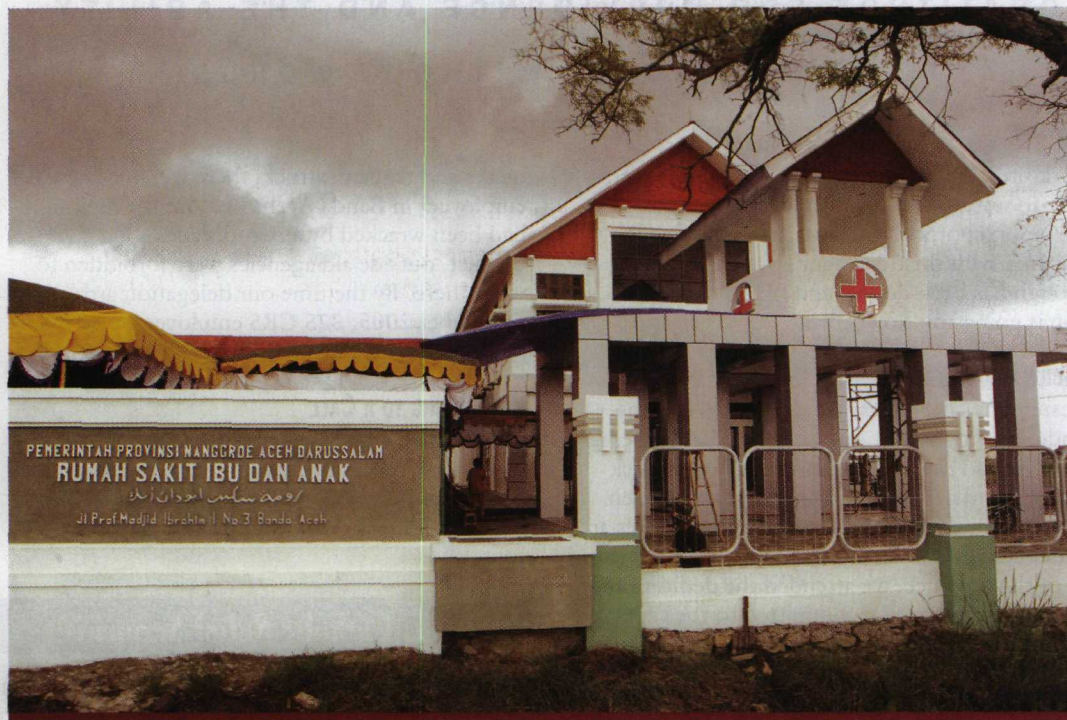
The newly constructed Banda Aceh Women and Children's Hospital.
